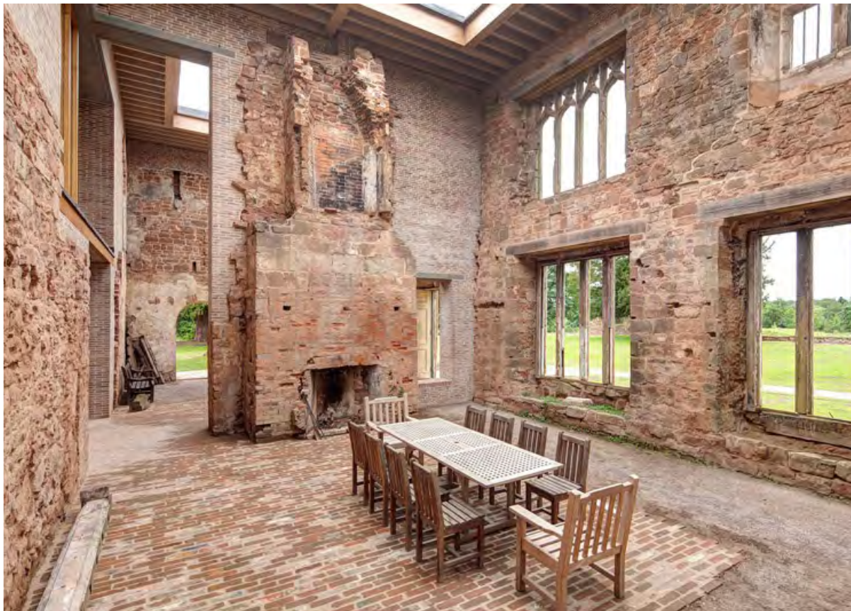
Astley Castle Renovation. Warwickshire. Witherford Watson Mann.
